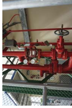
Pictures of PM Alarm Valve of Fire Sprinkler Systems
