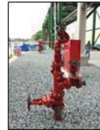
● Fire Hydrant with Monitor
